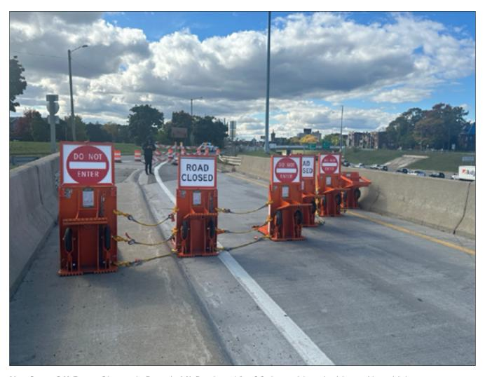
**Use Case:** Off-Ramp Closure in Detroit, MI. Deployed for 90 days with no incidents. No vehicle access. Replaced Type 3 barriers and orange barrels.
